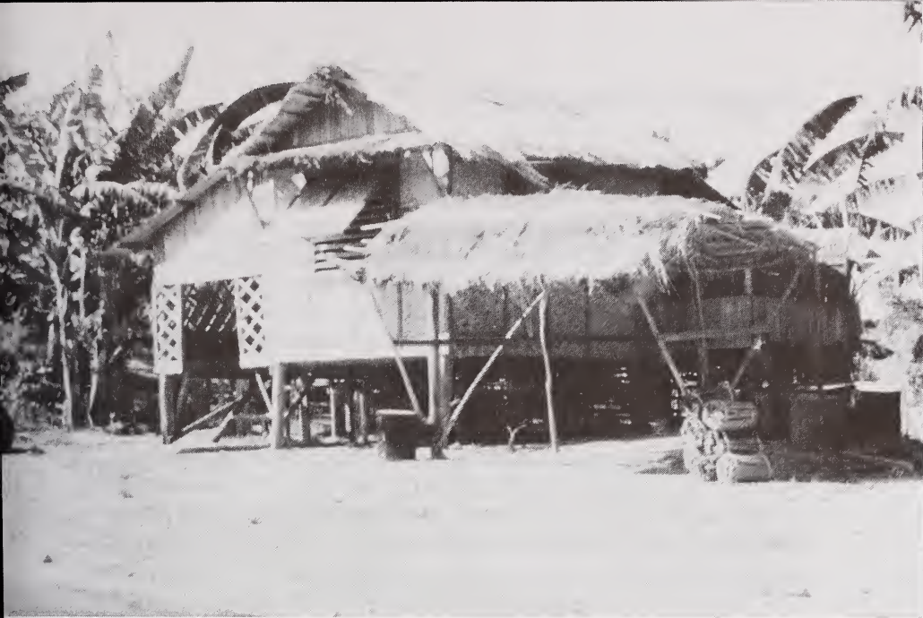
Typical rural Philippine nipa house, constructed of locally available bamboo and nipa-leaf thatching Courtesy Patricia V. Dolan
